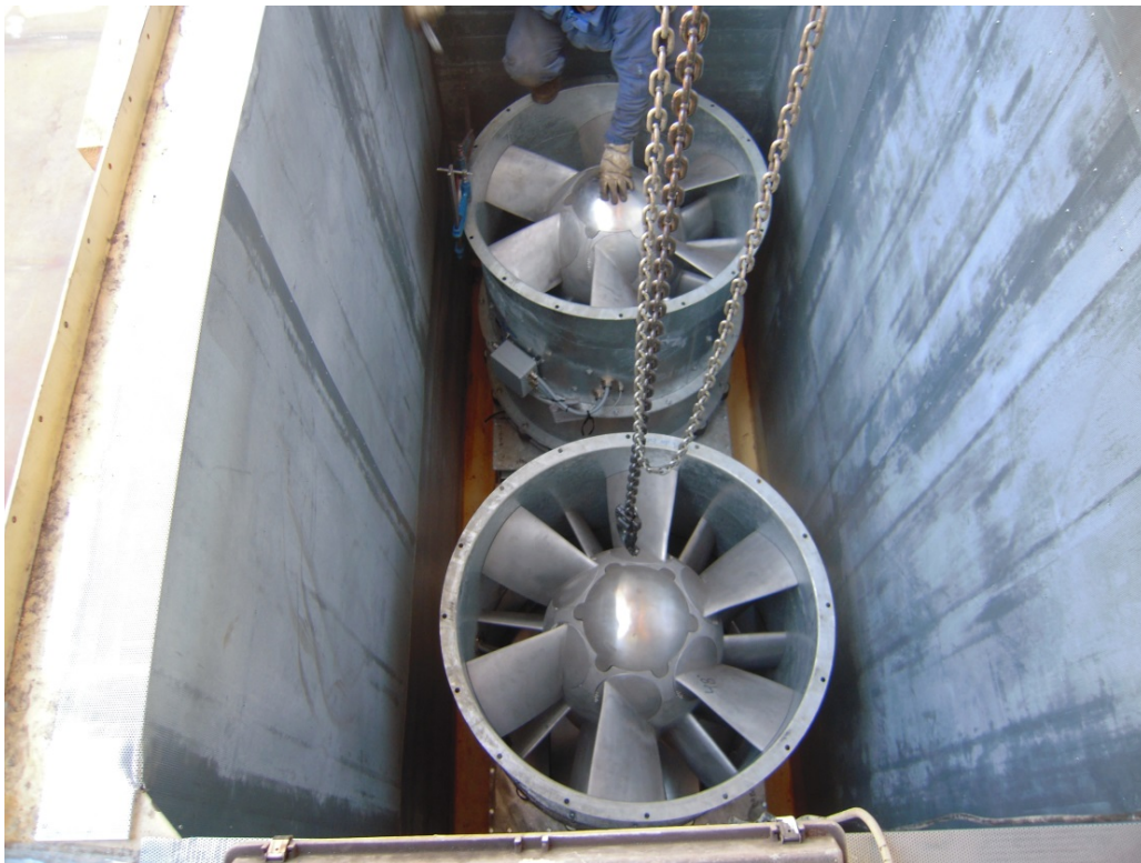
Engine room ventilation fans installed
