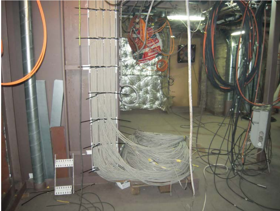
Cat 7 cable - LAN distribution on Main dk.
