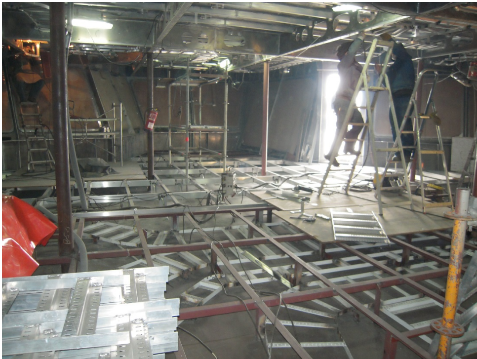
Wheelhouse – raised floor and cable trays in progress – Consoles are ready with the equipment mounted at KM in Vigo.
