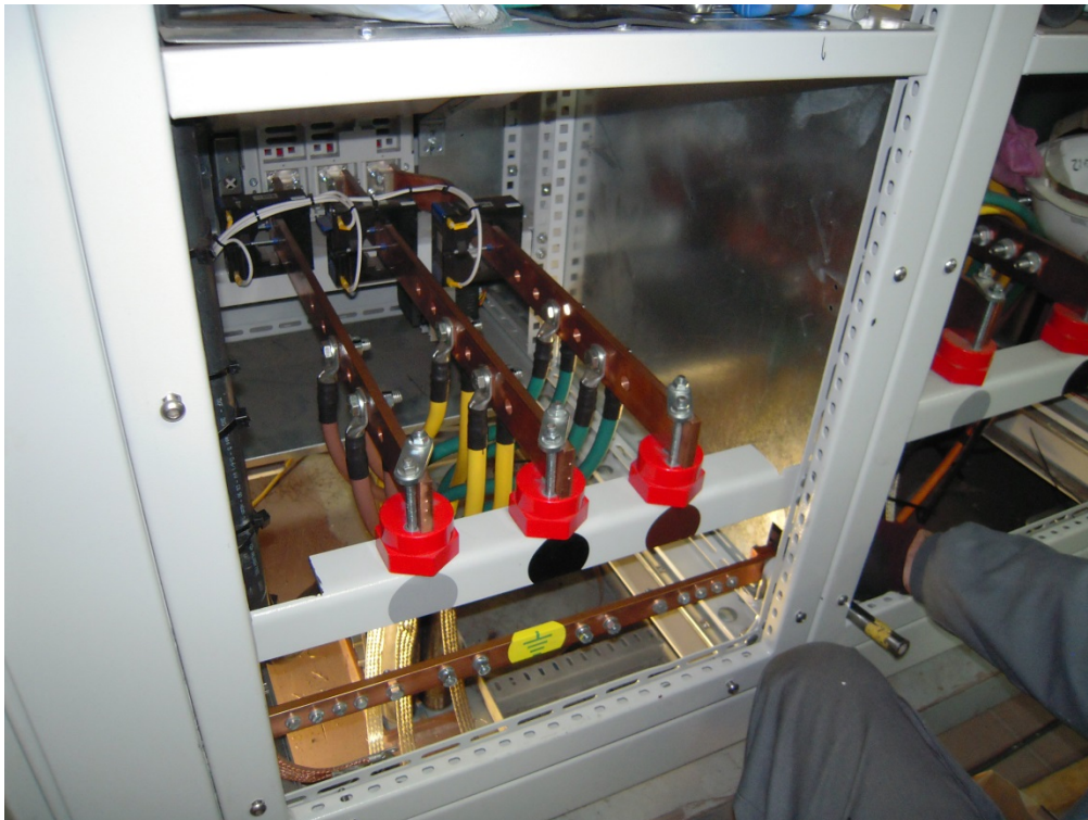
Termination in main switchboard
