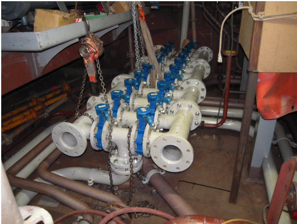
Fuel oil system - manifold and piping
