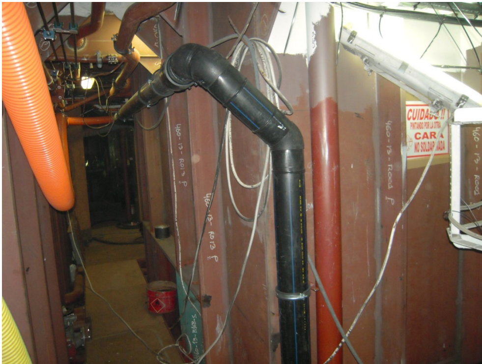
Clean seawater piping started
