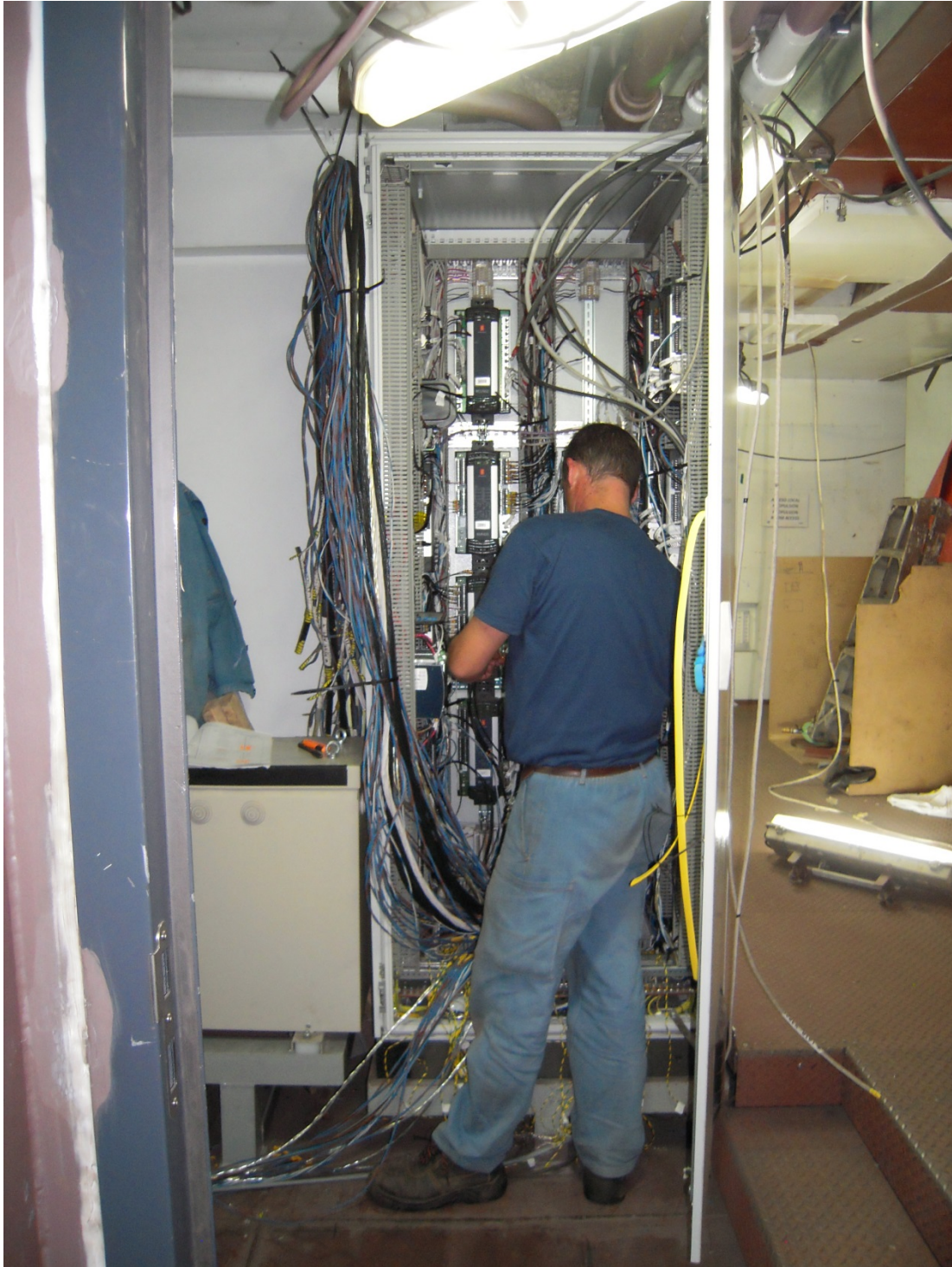
Termination in IAS (Integrated Alarm System) cabinets
